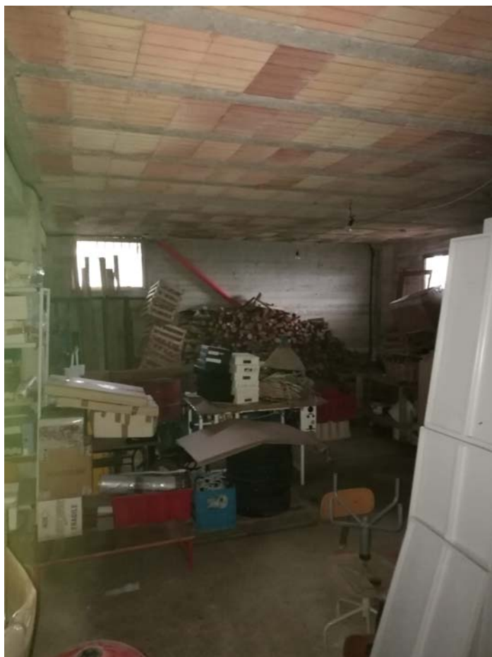
- Garage piano seminterrato
