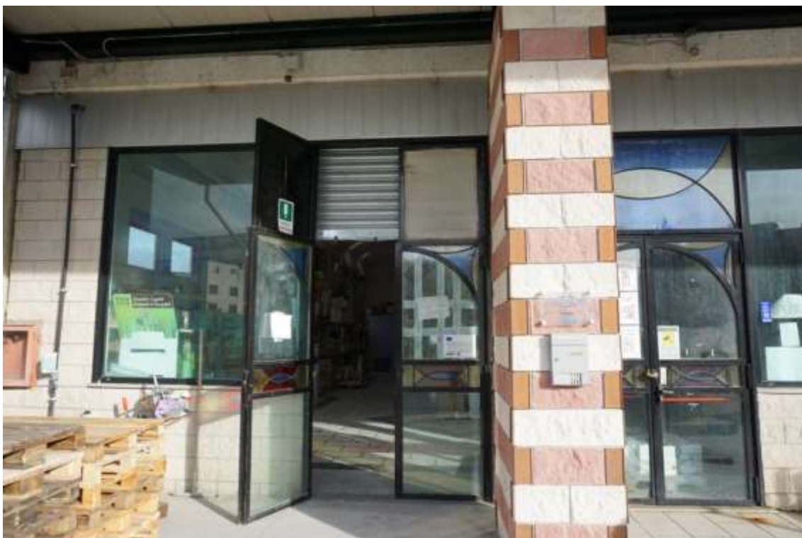
Fig.15 – Vista porte d’ingresso sub.18 (C1)
